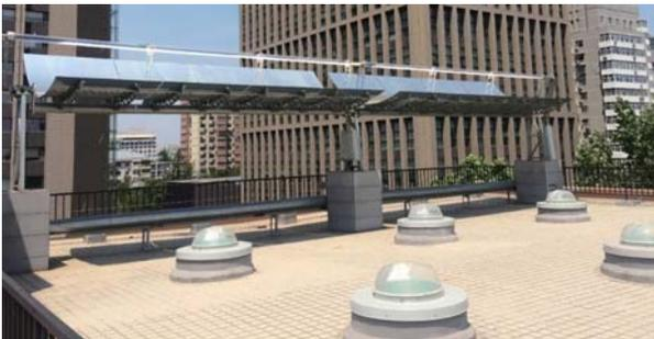
Figure 14 High temperature solar collector
