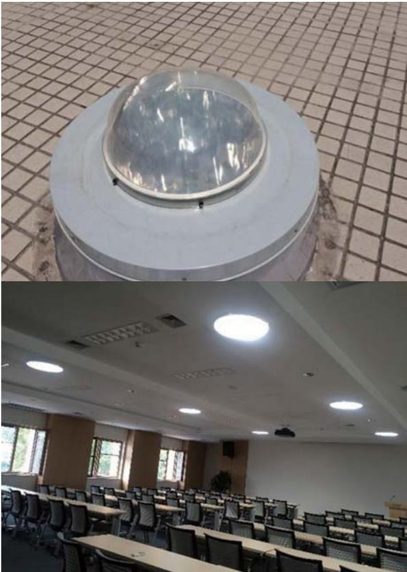
**Figure 9** Solar tubes (outside and inside)
