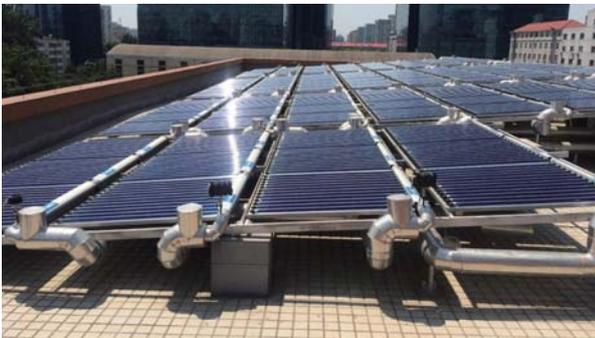
Figure 15 Median-temperature solar collector
