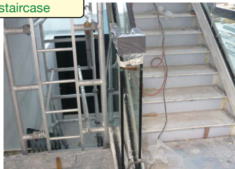
Addition of staircase
