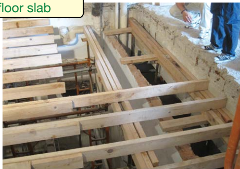
Alteration of floor slab
