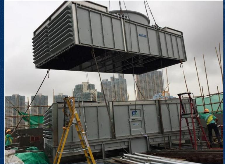
Module hoisted by tower crane, loading capacity was checked and confirmed in early stage
