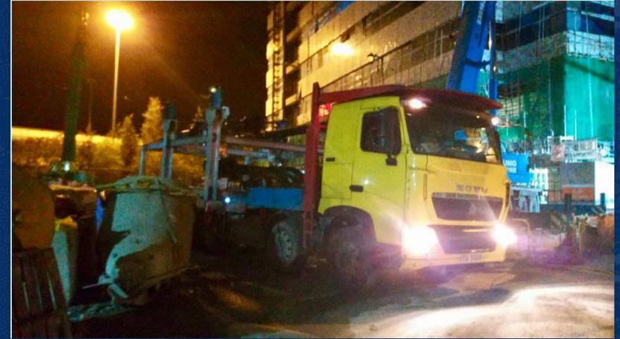
Mid-night delivery of modules due to the allowable lorry width for daytime traffic (3500mm)
