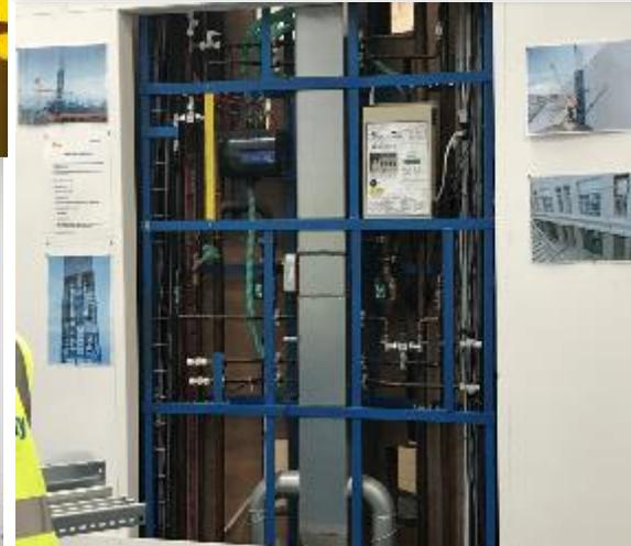
Prefab vertical riser module with catwalk
