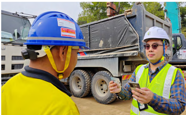
The Inspection and Enforcement Team conducted inspection at construction site
