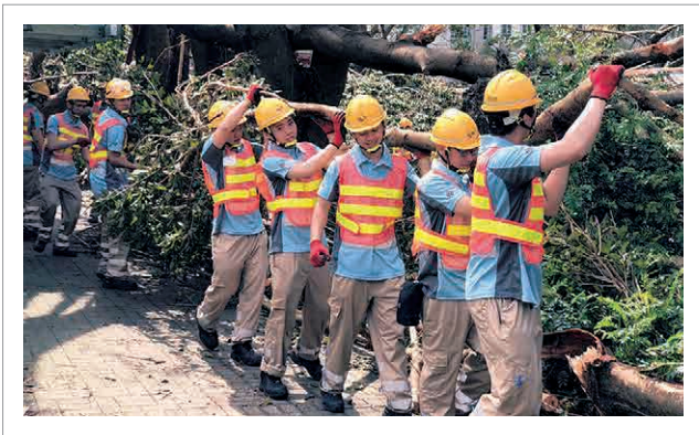
Post-typhoon relief and recovery work 風災善後工作
