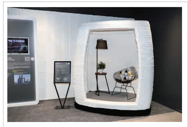
3D Printed Structure 3D打印建築結構
