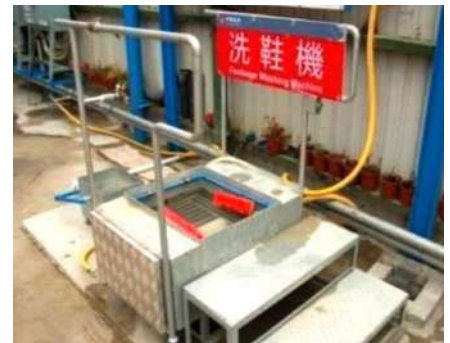
Shoes Cleansing Facility
