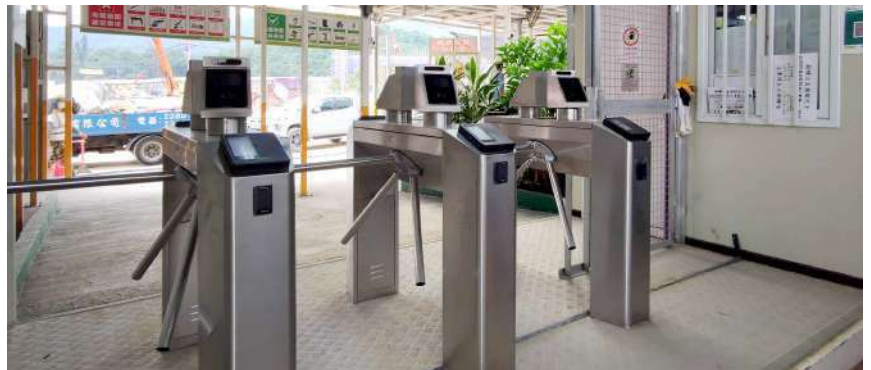
Set up the covered queuing area and an adequate number of gates with card reading devices
