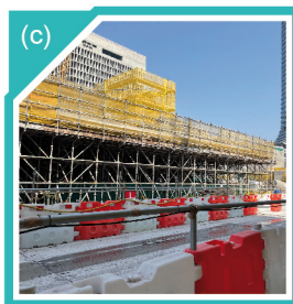
Water-filled barriers (Traffic management)
