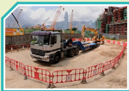
Figure 6 - Examples of Good Practices of Barricading Fatal Zone
