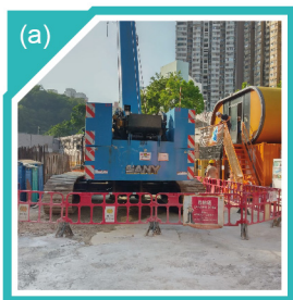
Interlocking red plastic barriers (Fatal zone management)
