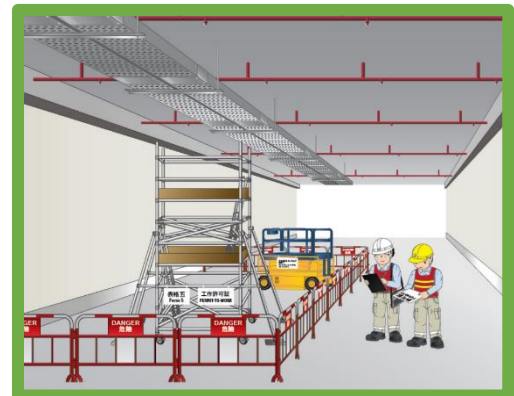
Suitable working platforms (e.g. power-operated elevating work platform or metal scaffolds) should be provided and used for working at height
