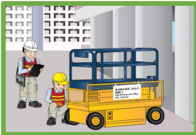
A MEWP with its associated critical parts should be regularly inspected, tested, and properly maintained in accordance with the manufacturer's instructions
