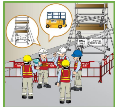
Suitable working platforms should be provided and used for working at height (e.g. mobile elevating work platform or metal scaffolds)
