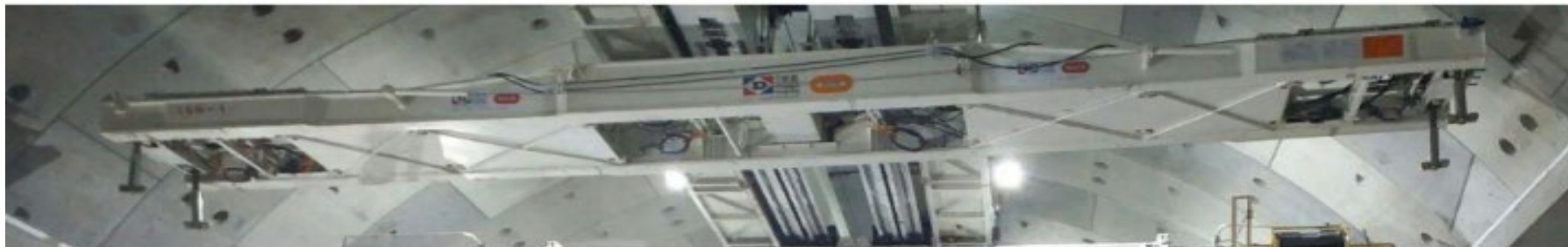
Lifting Spreader Beam after release of hammerhead support points
