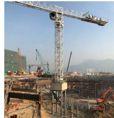
Tower Crane Base
