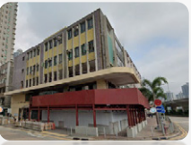
Price Edward Road West Demolition Works
