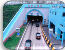
Tate's Cairn / Aberdeen Tunnel Maintenance Works
