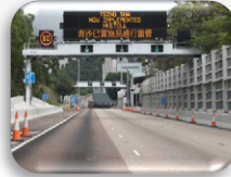
HKeToll Six Tunnels Maintenance Works
