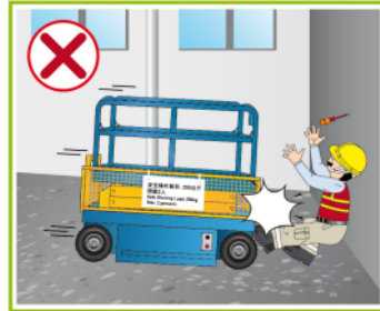
Do not park EWP on the slope
