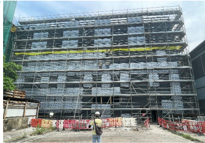
Step 2: Cladding installation
