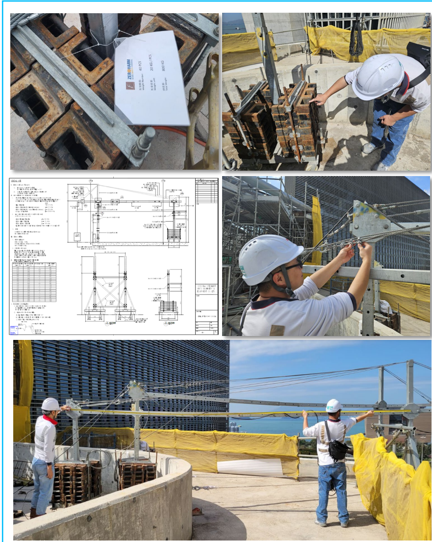
Checking of Gondola set up
