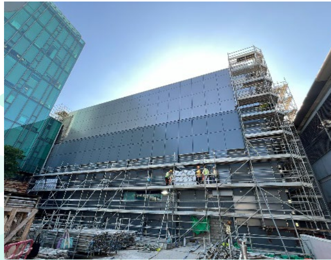
Step 4: Left out cladding installation
