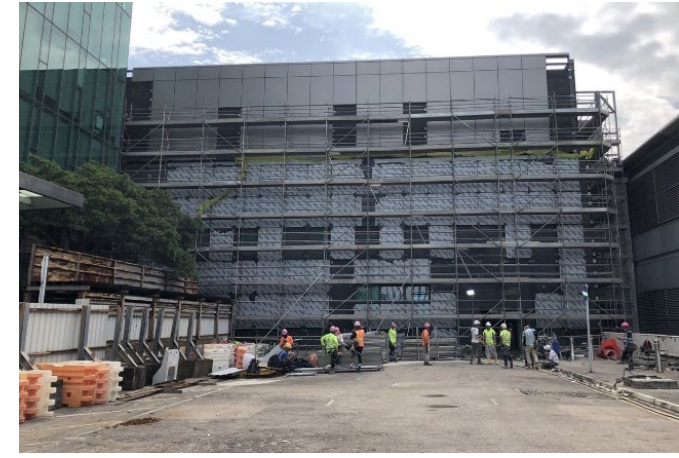
Step 3: Dismantle of scaffolding and removal of wall ties
