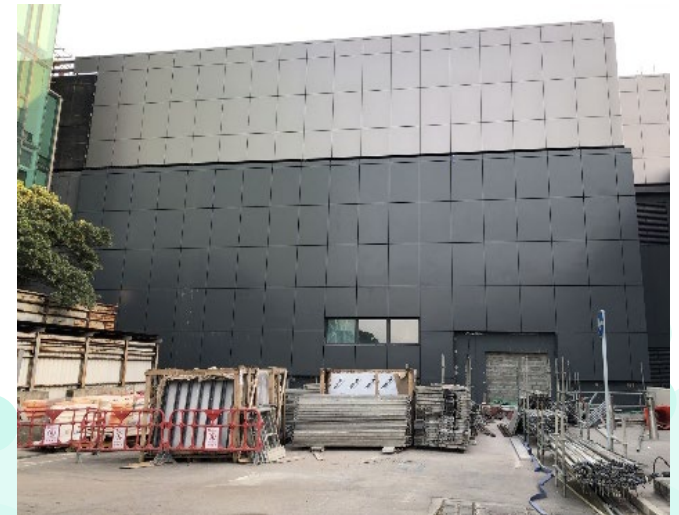
Step 5: Cladding installation completed
