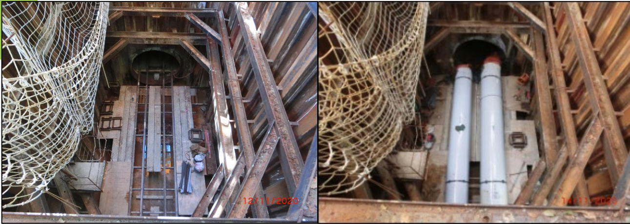
Aerial views of the launching pit (reference from other project)
