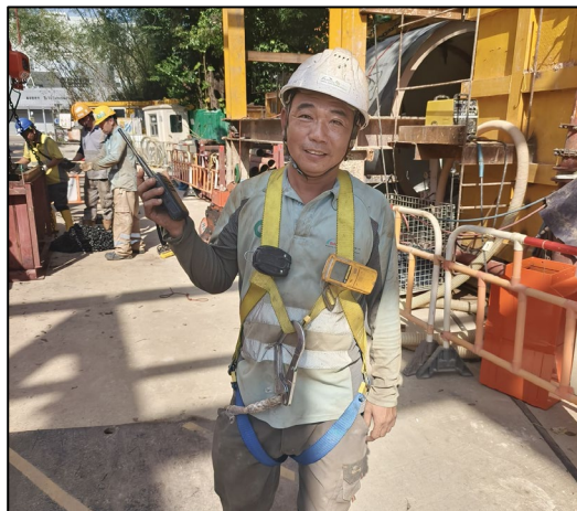
Workers' equipment before entry of confined space:
