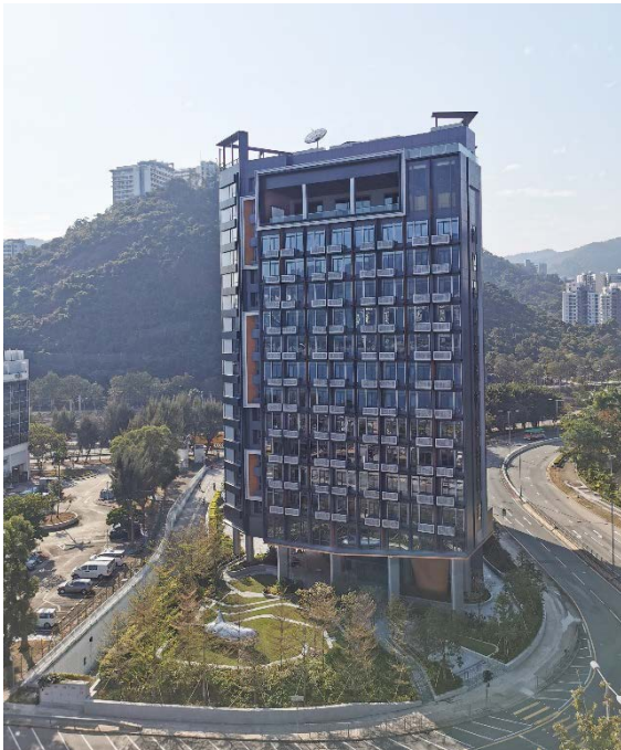
InnoCell is the first high-rise MiC building completed in Hong Kong, providing smart living and co-creation space for the I&T community at the Science Park
