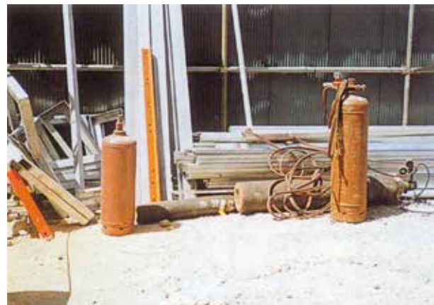
Mixed storage of empty & filled gas cylinders
