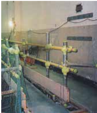
All the passageways are cleaned up; trash and waste have been properly removed
