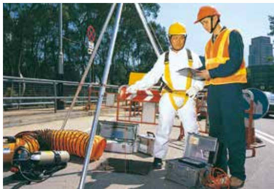
Testing the gases composition to make sure they meet the safety and health requirements
