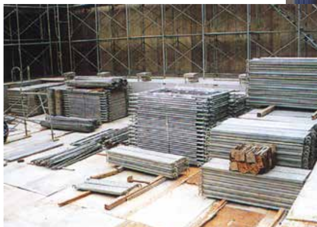
Materials are stored properly at site
