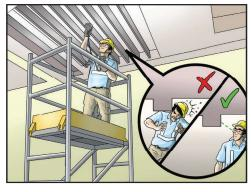
Workers should beware of overhead room and check for any obstruction to prevent accidental hit on the head before and during the use of working platforms. Safety helmets with chin straps should be used.
