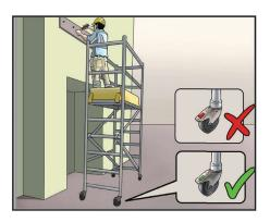
Ensure that all the castors are firmly locked in position while ascending/ descending and using a mobile working platform.
