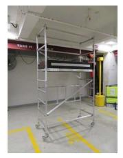
Figure 3: Mobile working platform
