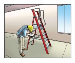
Before use, inspection (including visual check) of the light-duty working platforms according to the safety checklist provided by the supplier or other equivalent safety checklist should be conducted.
